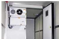
20ft Dual Zone Unit Chiller / Freezer 6,050 x 2,440 x 2,890 7,500 7,500 15,000
